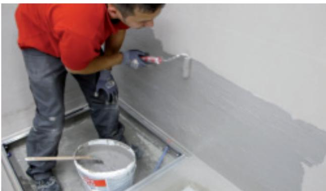
**4** To waterproof surfaces, apply Sopro FDF thickly to substrate using lambswool roller or finishing trowel, taking care to avoid pore formation. Apply second coat in a different colour when first coat has achieved adequate strength. Tile covering may be applied using flexible thin-bed adhesive (e.g. Sopro FF 450) when second coat has set.
