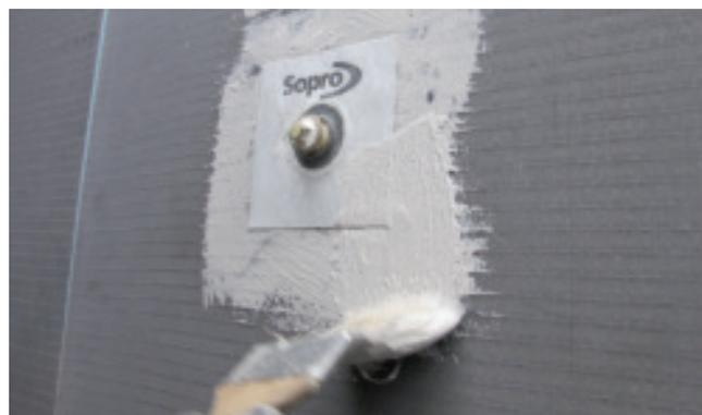
**2** Push Sopro DMW 090 sealing collar for walls over pipe end.
