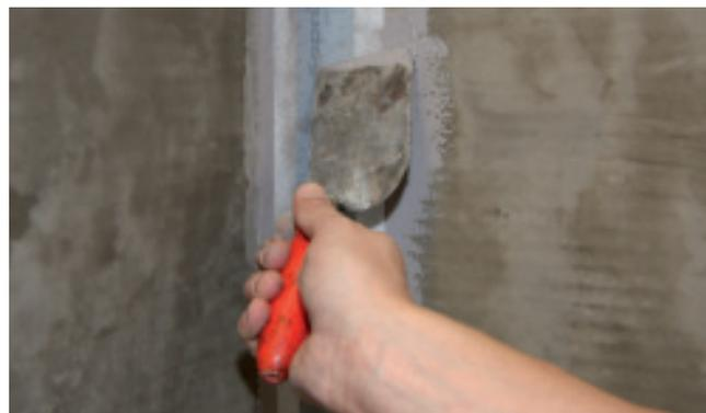
**1** First seal corners using preformed Sopro DE 014/015 sealing tape units, angles and wall/floor joints using Sopro DB 438 sealing tape. To do this, first apply Sopro FDF to primed substrate, place and embed sealing tape, and thickly overcoat nonwoven edge with Sopro FDF using brush or spatula.
